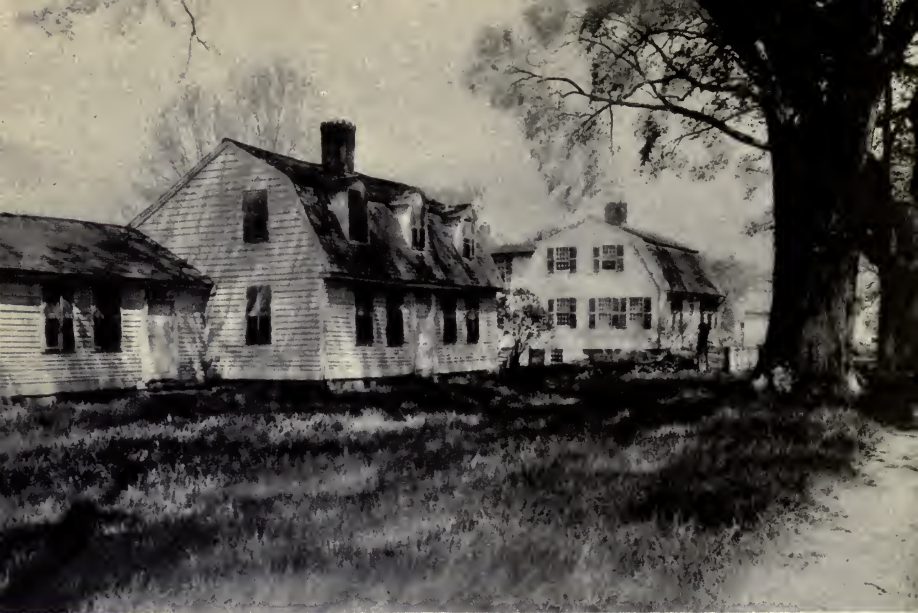
GAMBREL ROOFS, PLAINFIELD
